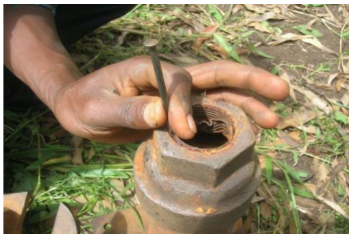
(c) Corroded pipe snapped off India Mark II cylinder in Uganda (old pipe threads being carefully peeled out to salvage cylinder) Source: Larry Bentley.
